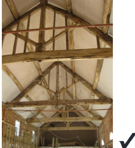
Fig 15: Original roof structure retained
