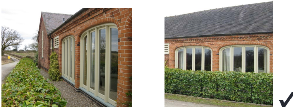
Fig 7: Large barn doorways with full height glazing
