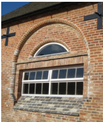
Fig 6: Example of sympathetic materials being used and existing openings being glazed. (NB. For this type of opening an inward opening hopper style window should be used instead of top-hung opening lights)
