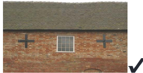
Fig 5: New window inserted in existing opening
