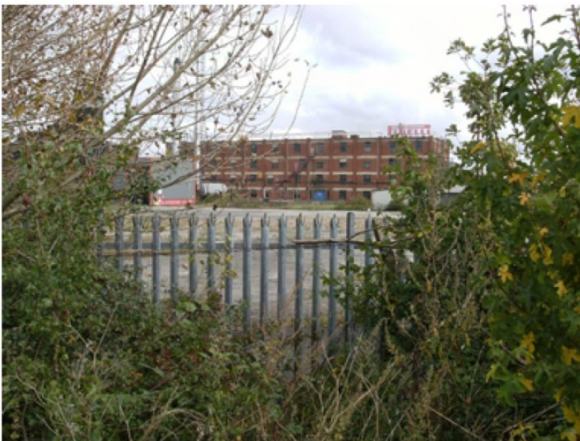
View of the Beech Avenue site from canal tow path
