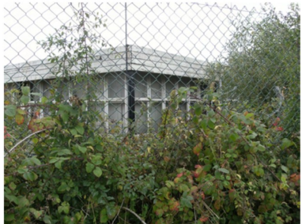
View of the Beech Avenue site from canal tow path
