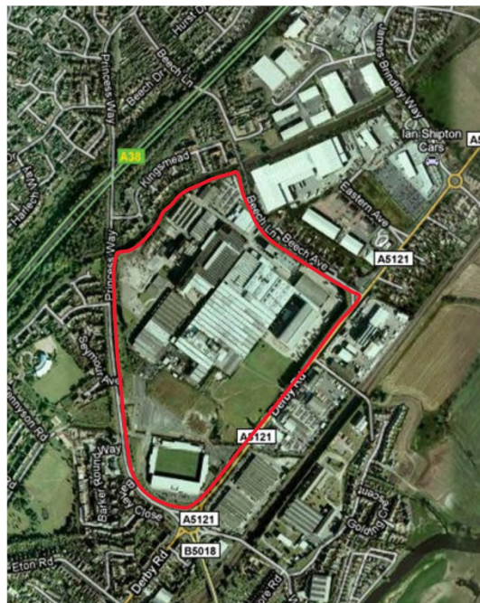
Aerial view of site
