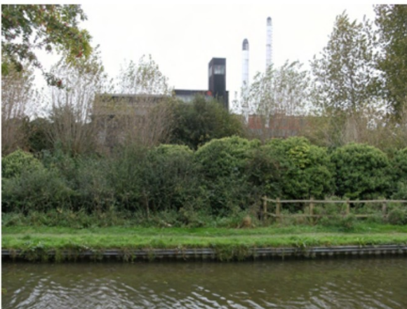
View of the Beech Avenue site from Kingsmead residential
