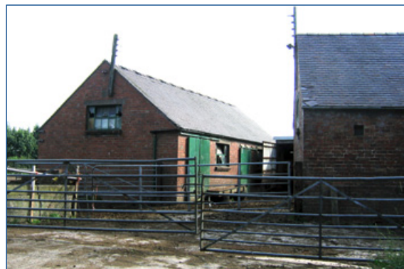
The supply of liquid milk was of prime importance from the late 19th century, and in the 1930s regulations led to the introduction of new stalling, windows and dairies (as here) to conform to hygiene regulations.
