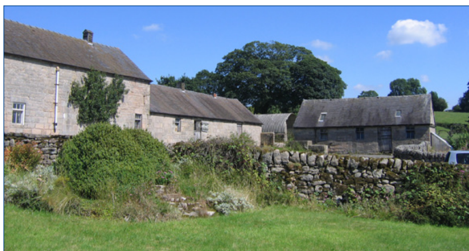
A loose courtyard plan with working buildings to two sides of the yard, with a barn and cattle housing on the left and a cowhouse on the right.
