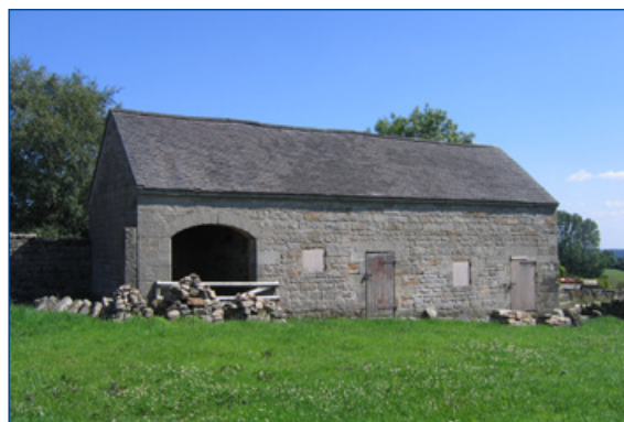
A large field barn sited in a paddock on the edge of Marsh Lane, Stanton.
