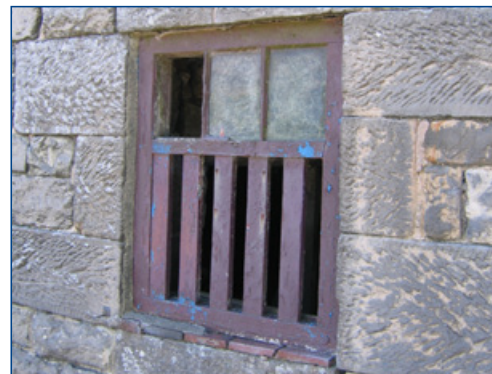
A window with hit-and-miss ventilators
