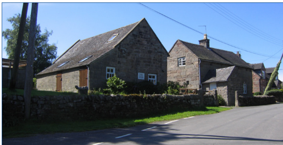
A small loose courtyard in the upland hamlet of Wootton with one working building – a combined barn and animal housing with additional housing for cattle in the rear lean-to.
