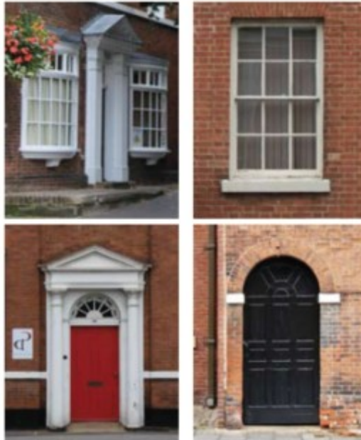
Windows and doors
