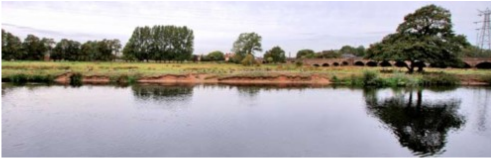
View looking west across the Broad Holme to the site with Burton Bridge on the right
