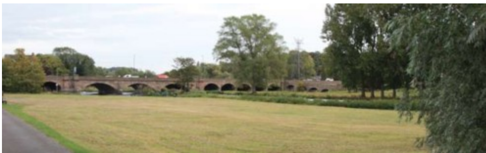
View looking north east from the Leisure Centre to Burton Bridge
