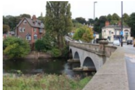
Burton Bridge looking east
