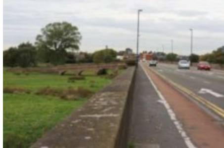
Burton Bridge looking west
