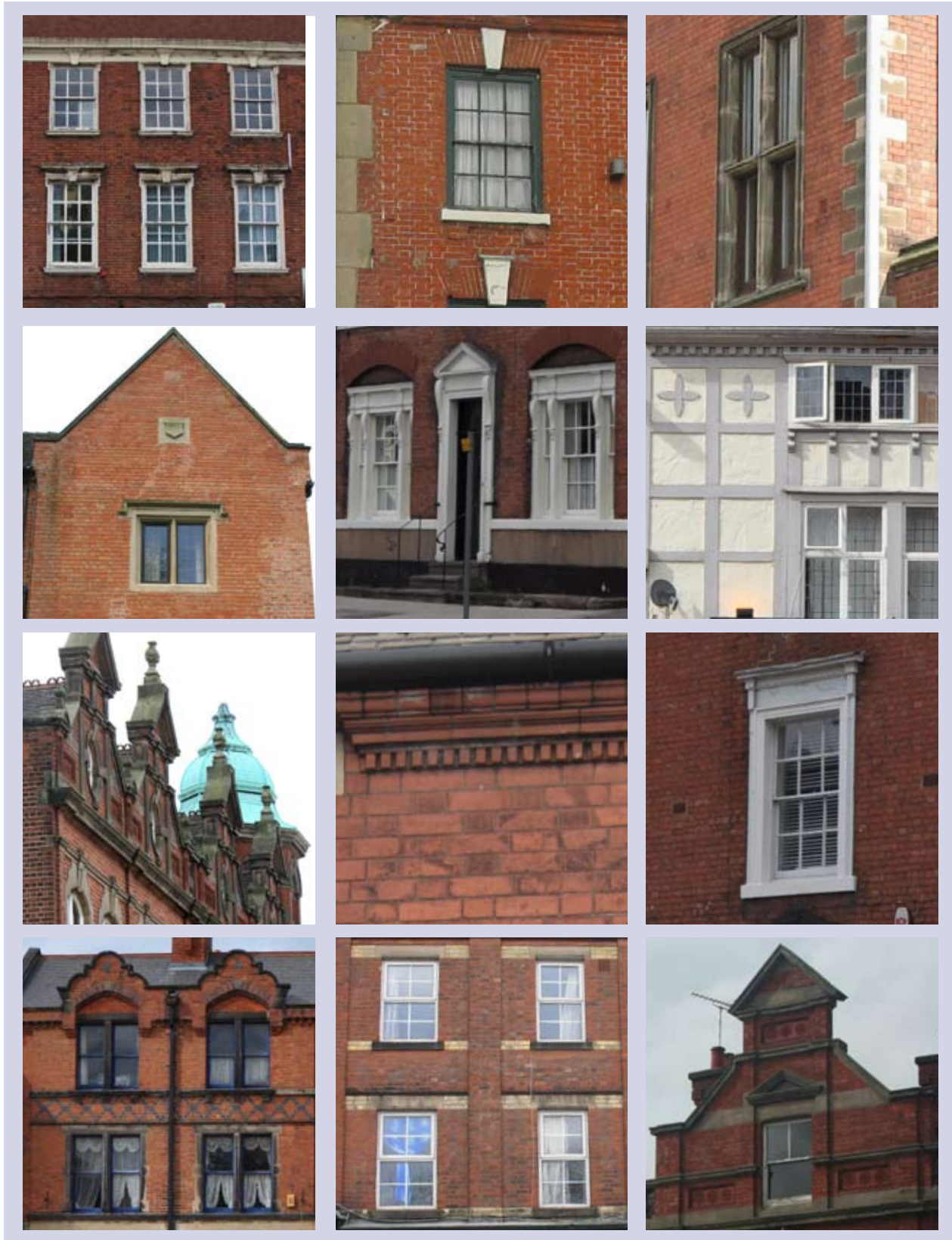
Some traditional architectural details in the town centre
