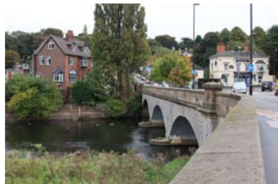
Burton Bridge looking east towards A511 / A444 junction
