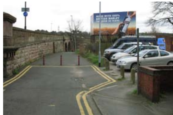
Pedestrian and cycle access off Bridge Street
