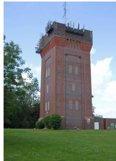
Winshill Water Tower
