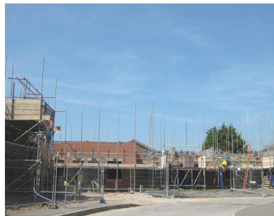
Construction at the old Renold Chain Site - Horninglow Road, Burton
