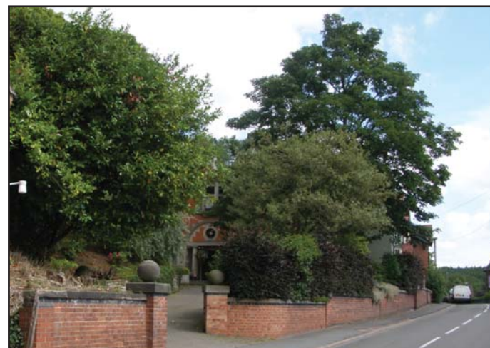
Red brick wall to Croft House
