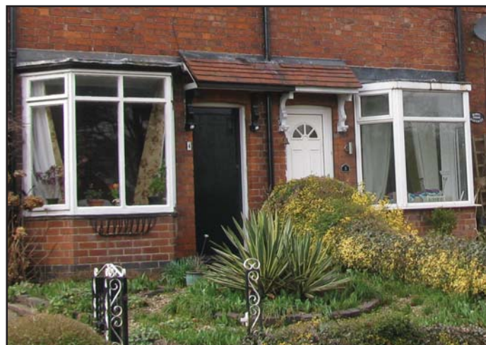
Replacement windows at Robinhood cottages
