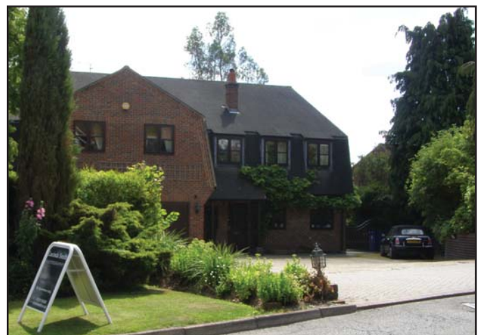
Brookfield House, Main Street
