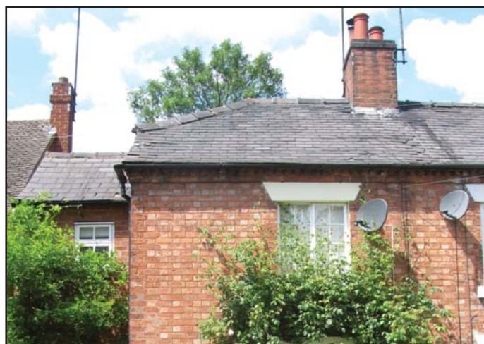
Hipped roof, New Row cottages
