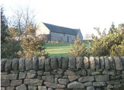
17: Semi formal dry-stone walling with rounded coping stones
