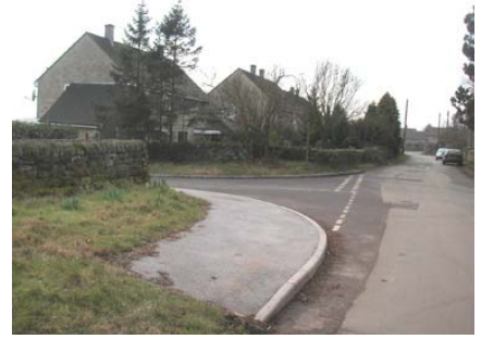
48: No need for this wide sweep of tarmac, grass would improve the surface appearance
