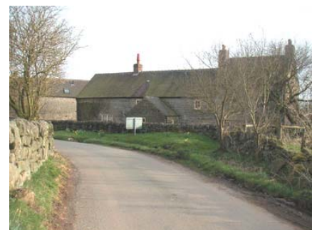
34: Containment and enclosure at the lane turn, at the eastern end of the village
