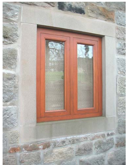
41: Although the colour of this window is still bright it will mellow to blend and the neat flush section is sympathetic to the vernacular and works well in terms of weathering
