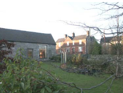
18: Imaginative barn conversions contrast with the curiously brick fronted Freba / Woodbine Terrace
