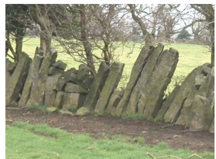
5: Stone slab walls
