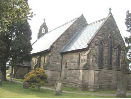
23: Slate roof details to the re-roofed St. Mary's Church
