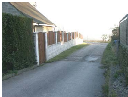
47: Mechanical appearance of the wall and fence on an important gap lane / view
