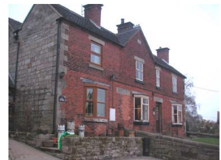
21: Unexpected reversal of material from stone to brick; the properties would improve with some thoughtful redesign and matching of the windows
