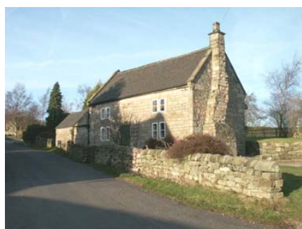
39: Parapet gables, and external gable end stack, small casement windows – an attractive vernacular
