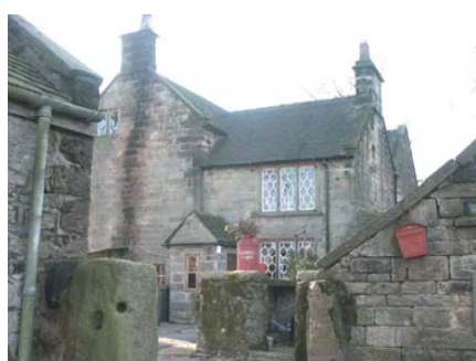
38: Paddock Farmhouse – the symmetrical main frontage is however, turned away towards the fields – this would be reversed in the centre of a town or village
