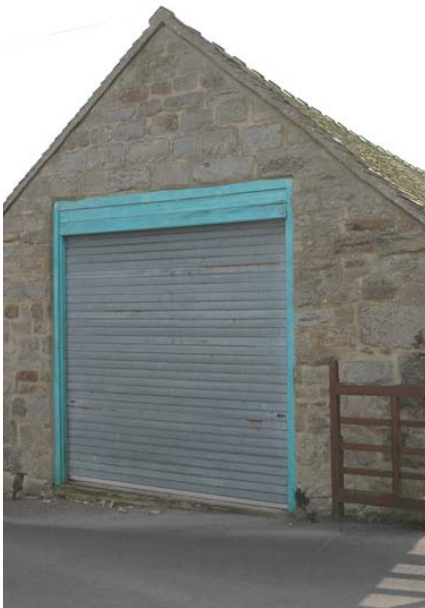
46: A dark colour for the door would reduce its impact on the nearby surroundings
