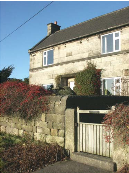
24: Note string – course and stone bracketed hood
