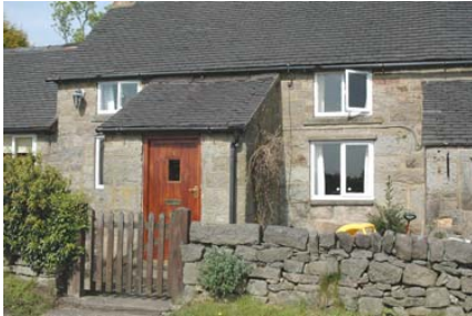
27: Simple casement windows – worthy of retention and copying
