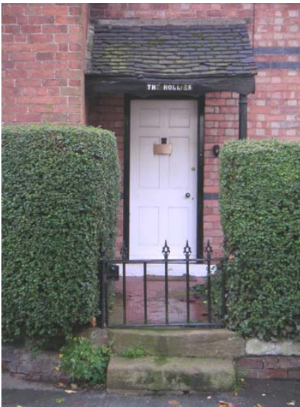
53: Old bracketed lean-to porch
