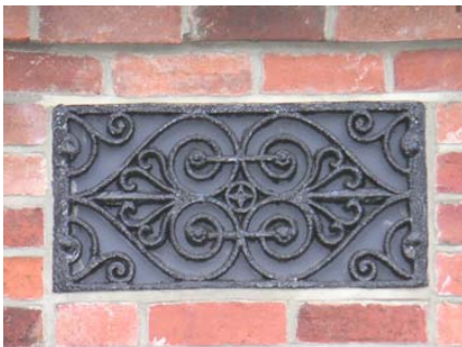
29: Cast-iron ventilator found in several parts of the village and in outlying farmsteads
