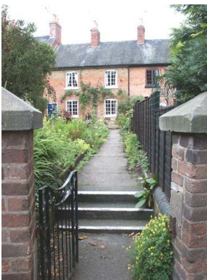
22: Gated path along raised gardens to cottages
