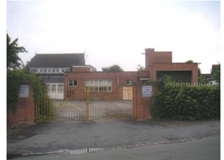
56: The extended set-back of the buildings and their design styles do not enhance the character or appearance of this otherwise intimate lane
