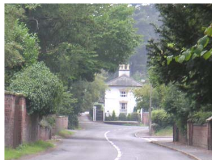
34: No:9 Church Road – listed lodge with railings
