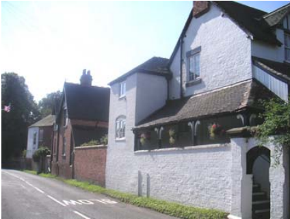
36: Attractive irregularity of massing and features on Church Road
