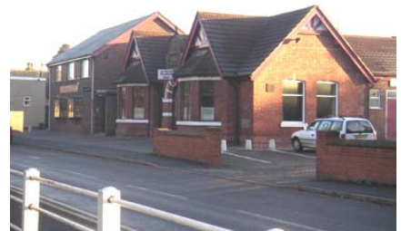
31: Rolleston Club – frontage
