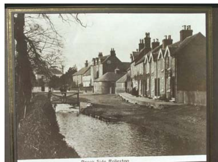
42: Brookside c 1900 with the 'Bull House' side building next to Brookside farm : now gone
