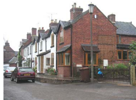
41: Cottages on raised pavement along Brookside
