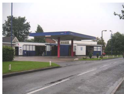
55: Prominent functional details that do not meld easily with the surroundings
