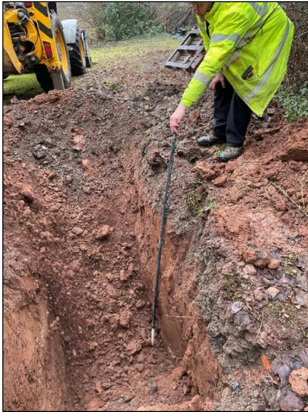
Figure 29. Installation of a dipwell – TP1.
