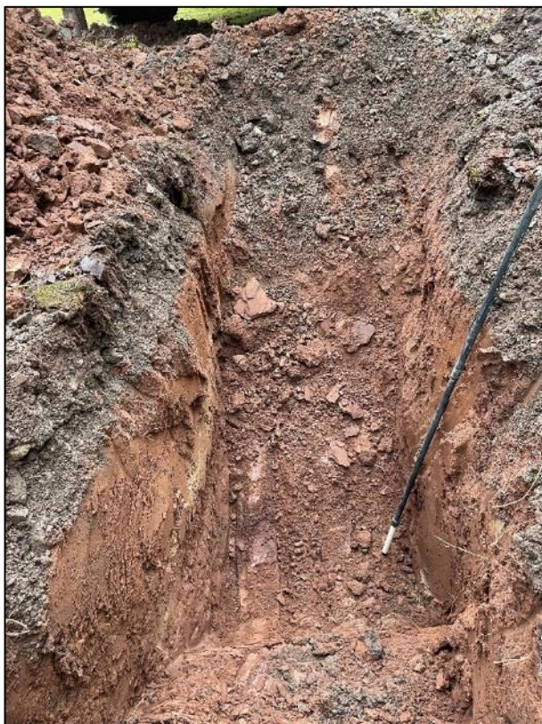
Figure 25. DOT Type 1 stone over SANDY SILT LOAM subsoil – TP1
