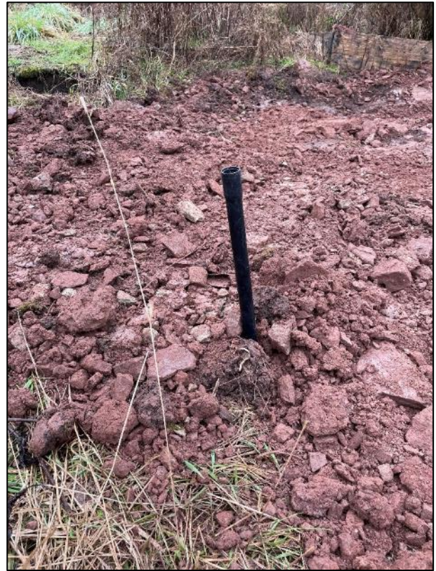
Figure 36. Dipwell installed TP2.
