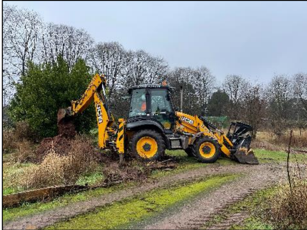
Figure 24. Digger used to excavate soil profile pits.
