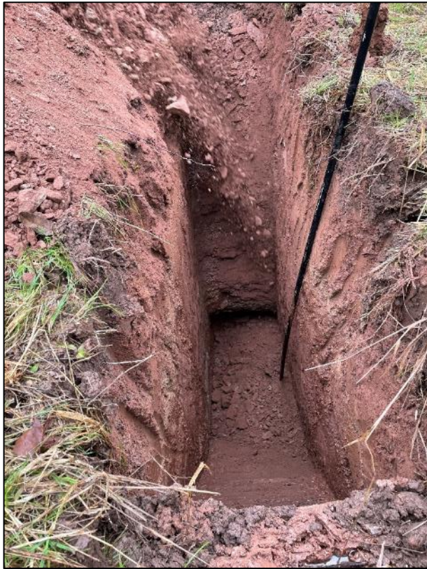
Figure 35. Dipwell installed TP2.
