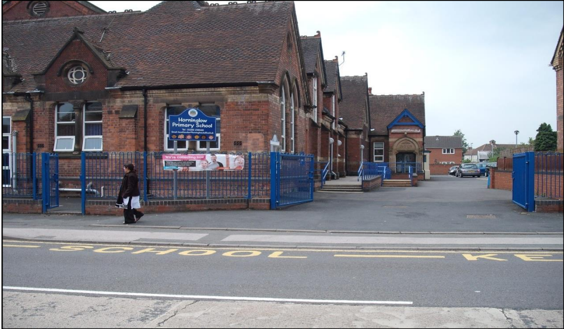
Horninglow Primary School
