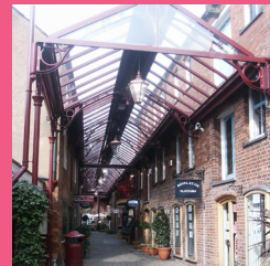
Retaining and reusing our valued structures
