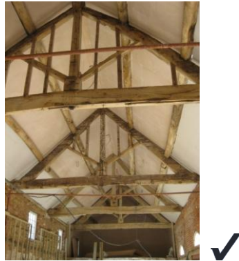
Fig 15: Original roof structure retained
