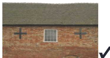
Fig 5: New window inserted in existing opening
