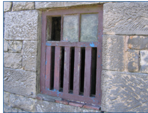
A window with hit-and-miss ventilators
