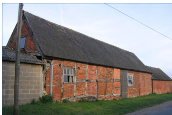
A threshing barn south of Yoxall, in a part of the southern half of the Middle Plateau and Valleys where smaller farmsteads remained into the 19th century. The square panel framing is a typical example of a distinctive carpentry tradition across the West Midlands.
