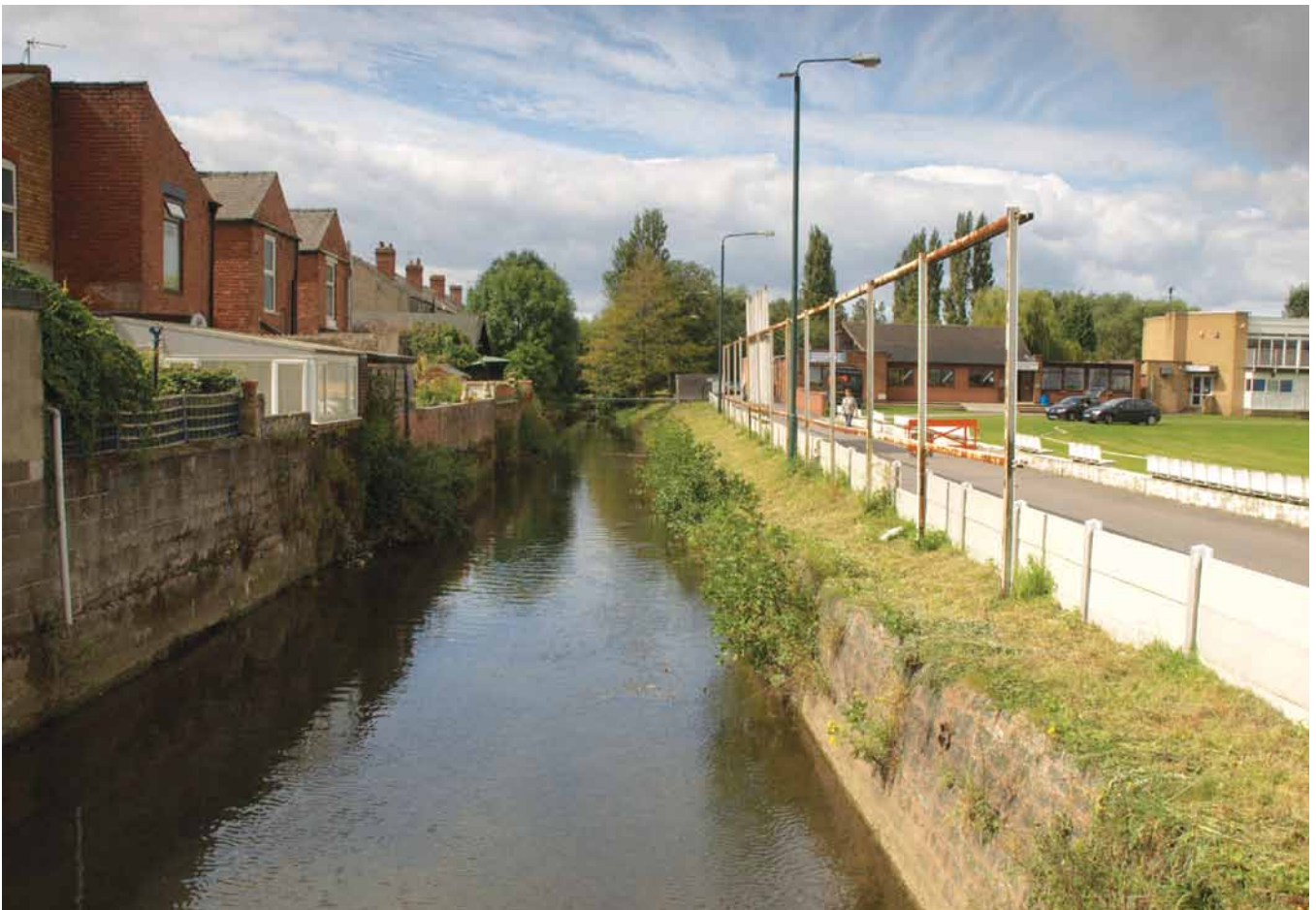
↑ Flood defences, River Ryton, Worksop
