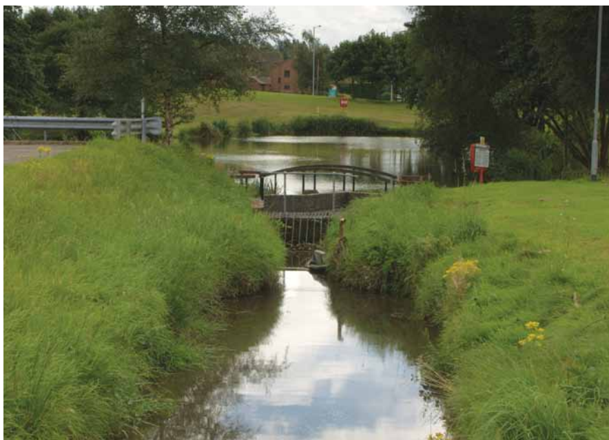
↑ River Churnet by-pass channel and balancing pond, Leek
