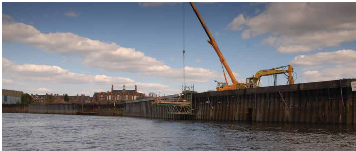
↑ Flood defences, Gainsborough
