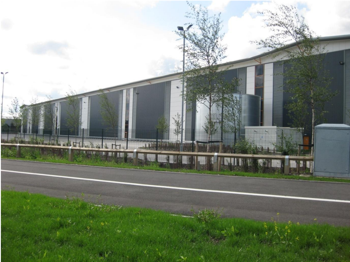
PHOTOGRAPH 1: CENTRUM WEST – A NEW BUILD DEVELOPMENT PROVIDING B1 AND B8 USES. CURRENTLY OCCUPIED BY PALLETFORCE DISTRIBUTION.
