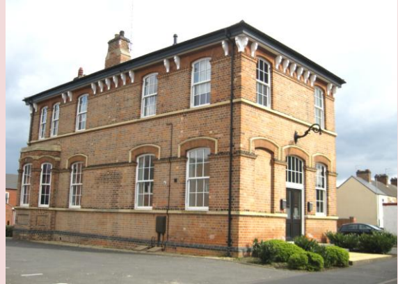
Converted Building within Clarence Street/ Anglesey Road Conservation Area
