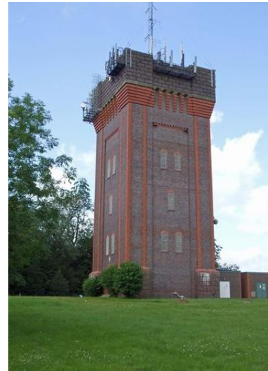
Winhill Water Tower
