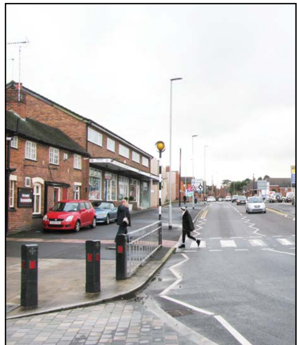
Parking on the pavement on Smithfield Road
