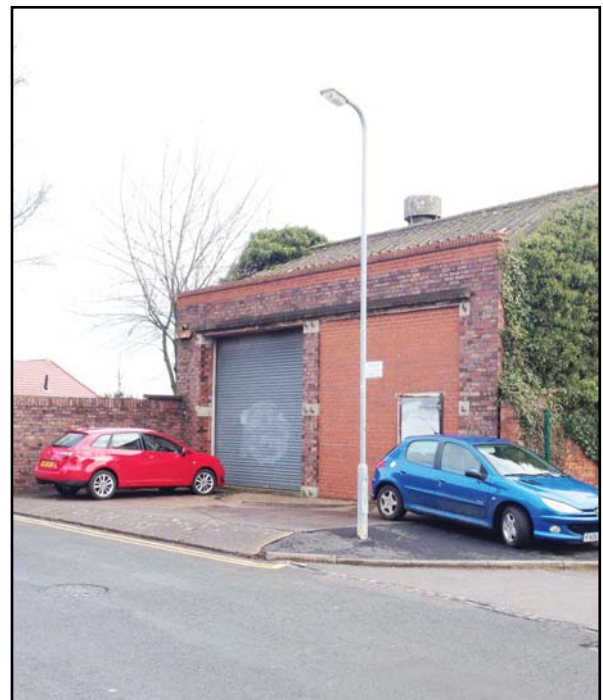
Potential brownfield site, Cockstubbles
